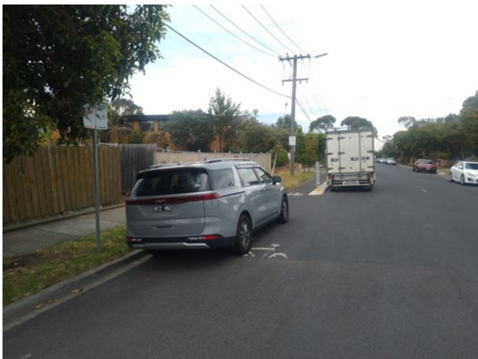
Figure 12: Protected bike lane abruptly ends into car parking spot (Footscray)
